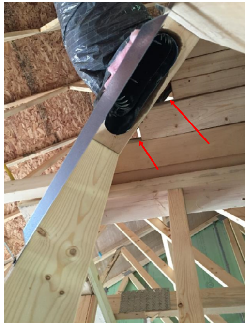
Connected to attic
